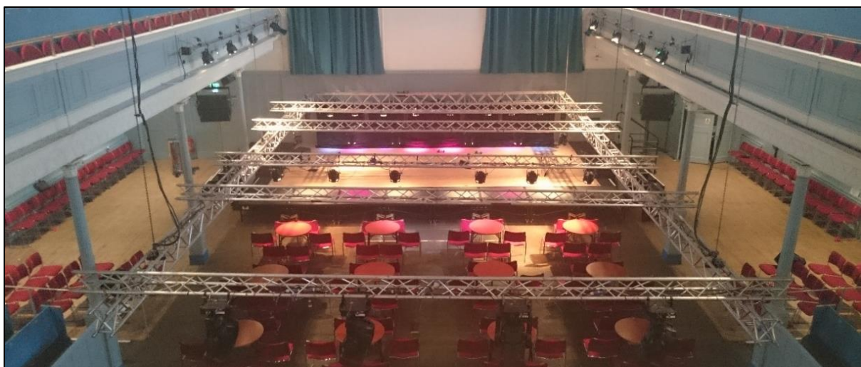
View of truss in lowered position.
