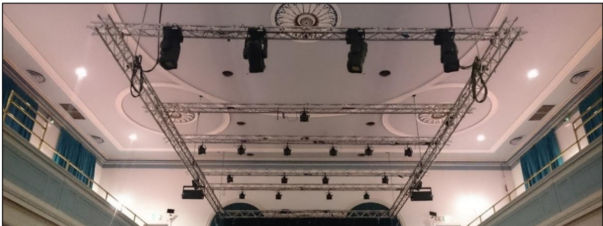
View of truss in raised position.
