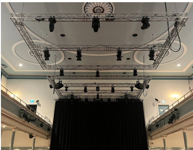
View of truss in raised position.
